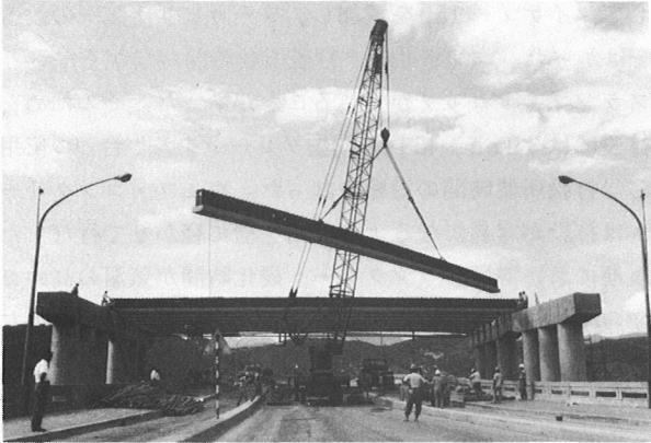
写真-7 Span=29.95m架設
