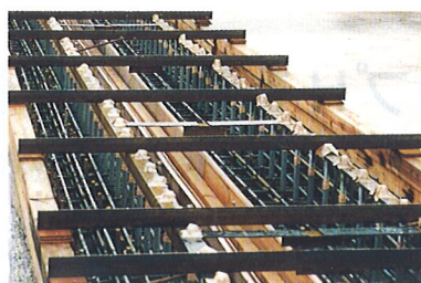
鉄筋鋼棒組立て
